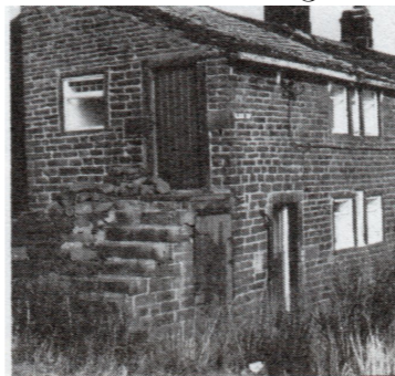
A taking-in door, at first floor level, at a handloom weaver's cottage in Yorkshire, showing the stone steps that gave access to the doors
